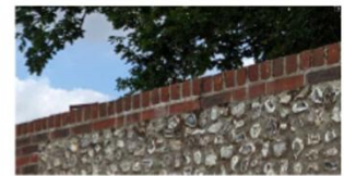
Flint wall with red brick coping
