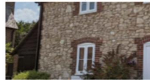
Local limestone and dark red brick reveals
