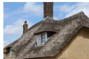
Half hipped thatched roof with hipped dormers
