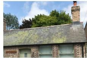
Gabled roof with grey slate tiles
