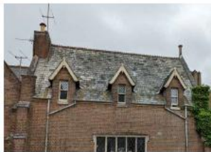
Pitched roof with dormers.
