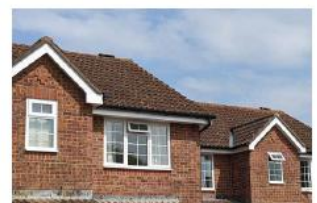
Clay tiles on cross gabled roof
