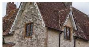
Rough ashlar wall with stone mullioned window
