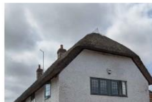
Half hipped thatched roof
