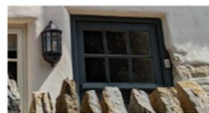
Casement windows (painted blue)
