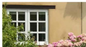
Modern casement windows
