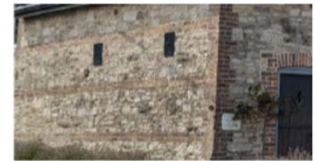
Local limestone and dark red brick reveals
